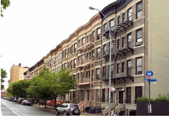
531-549 Bergen, looking west
